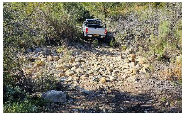
Typical example where stormwater infrastructure has either been blocked/damaged in need of repair, or where exposed rock through streambeds wash away repeatedly and which can be anchored instead with reno mattresses to reduce maintenance through regular flooding damage.
