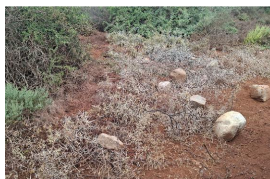
Figure 19: Example of area packed with large rocks and branches to support regrowth in an area where construction vehicles deviated from the designated turning and passing bays.
