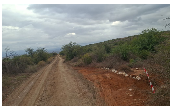
Figure 13: Example of temporary designated passing bay along narrow track to enable large construction vehicles to pass each other. Area must be clearly marked and rehabilitated once repair work is completed.
