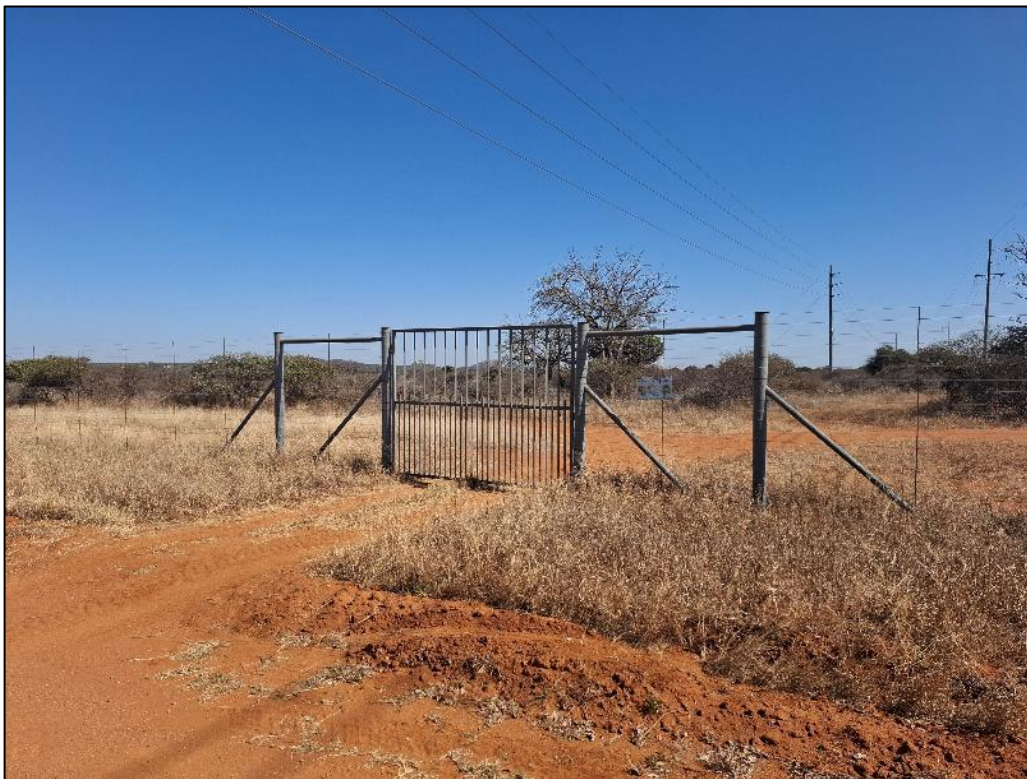
Photograph 3.9: Eskom transmission line corridor south of Tabor Solar PV Cluster site (OPHL Alternative 1)
