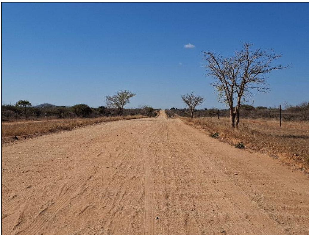
Photograph 3.4: View along Mogwadi/Bottelier Road looking west
