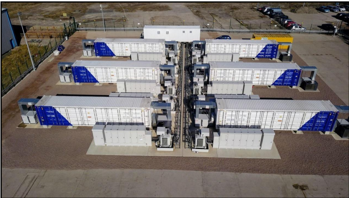
Photograph 1.2: Example of BESS located in storage containers
