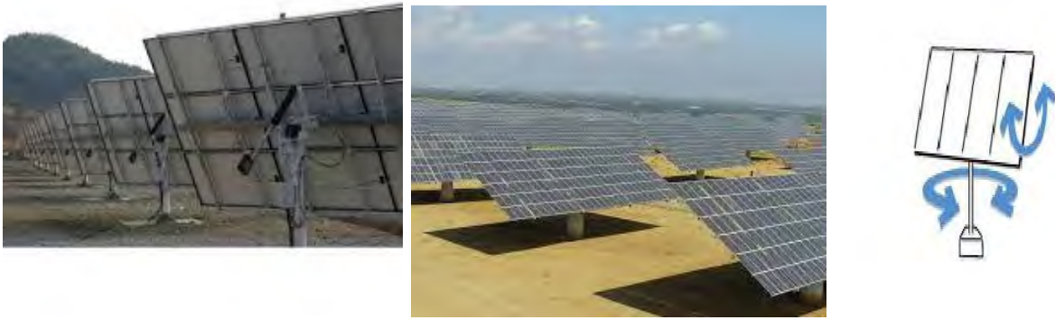
Figure 5: Examples of double axis PV tracking systems.
