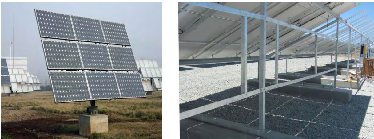
Figure 6: Examples single axis & fixed solar cast foundations.
