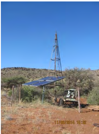
Figure 20: Solar pump and borehole.
