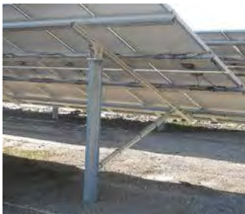
Figure 7: Typical rammed or screwed method of installation.
