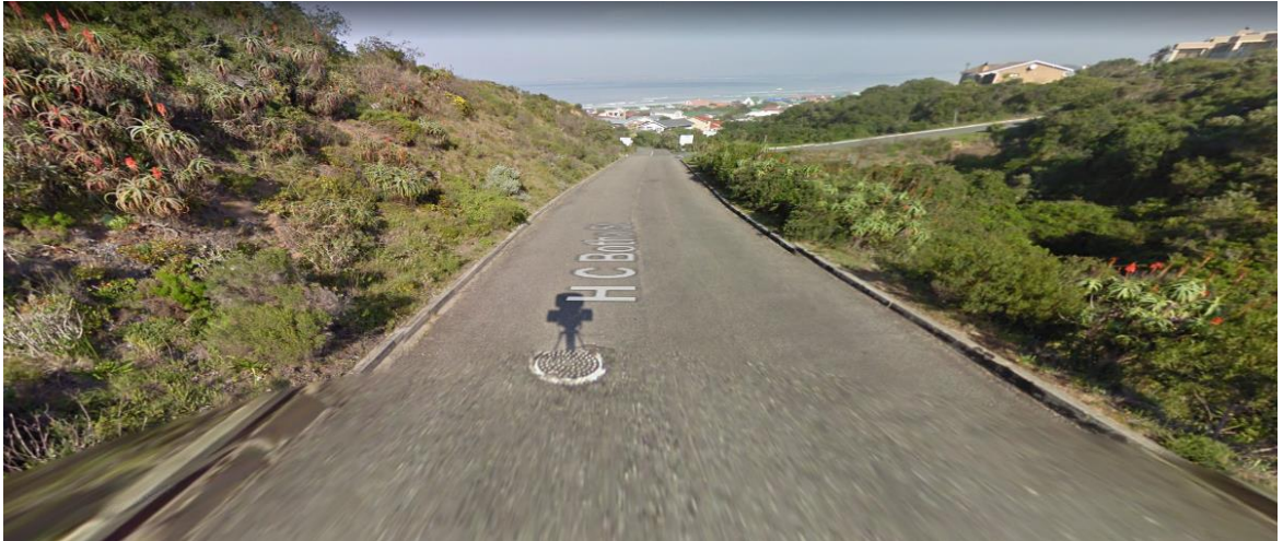
Figure 10: South-western view along HC Botha at the proposed access. Sight distance is excellent in both the horizontal and vertical alignments.
