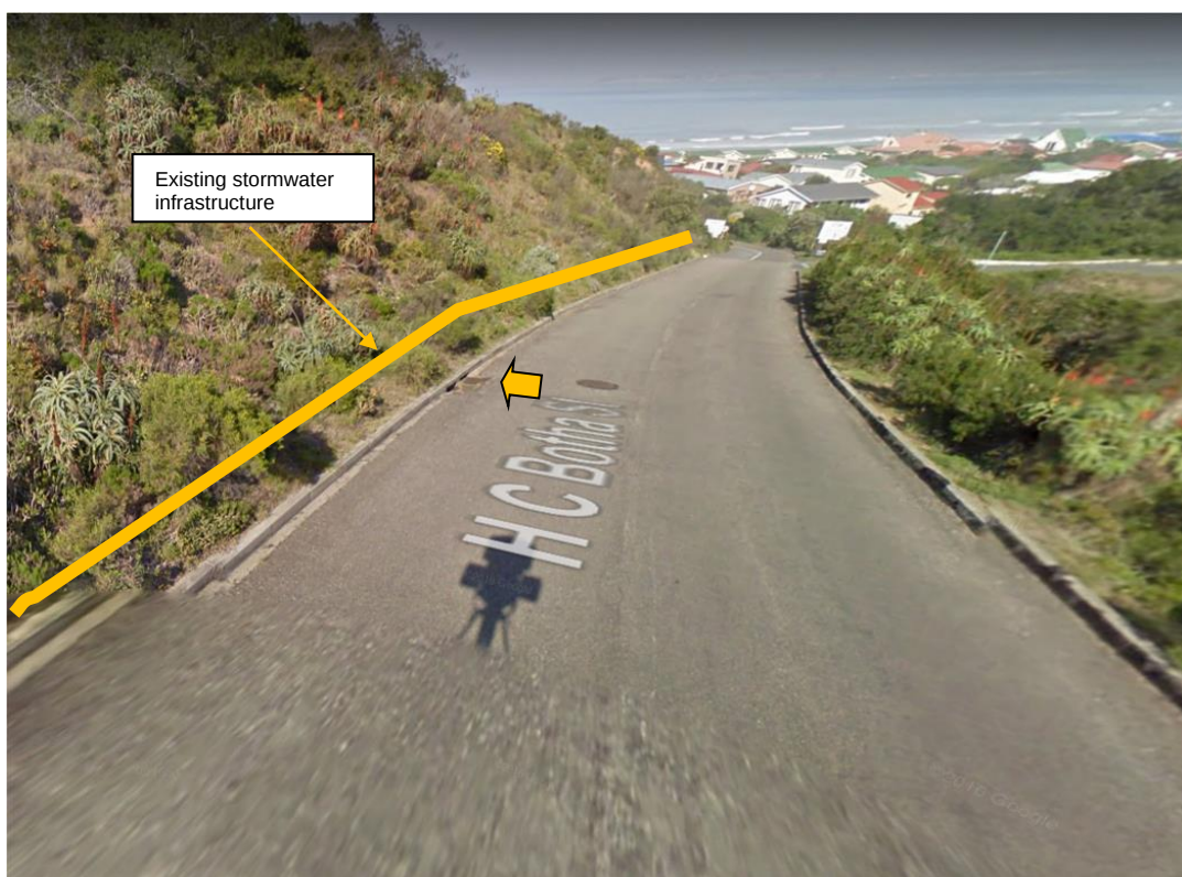
Figure 15: Existing stormwater inlet in HC Botha street south of the entrance to the proposed development.
