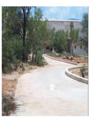
Figure 12 Completed cement surfaced road built with Hyson Cells
