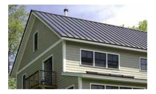
Figure 4 Typical klip-lok roof sheeting
