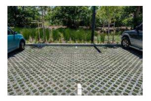
Figure 15 Pre-cast concrete grass blocks
