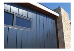
Figure 2 Typical fibre cement wall cladding
