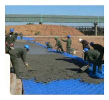
Figure 10 Hyson Cells filled with concrete
