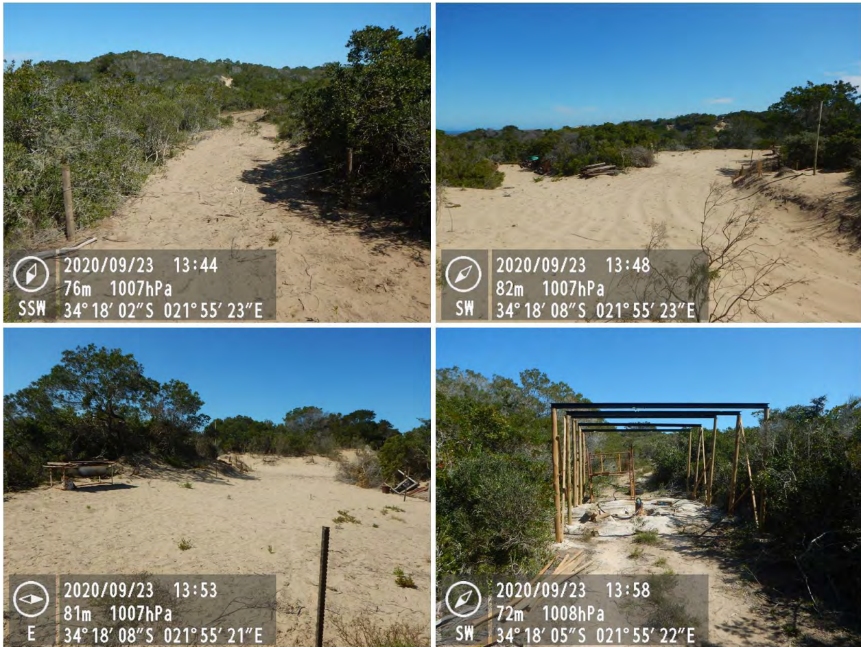
Figure 7. Examples of the affected environment along the access road and at the building footprint of the cottage (removed from plans) showing topography, vegetation cover and exposed dune sands. Metal fence droppers mark the footprint boundary points. The existing borehole is shown in the bottom right image. (A4 version on page 52)
