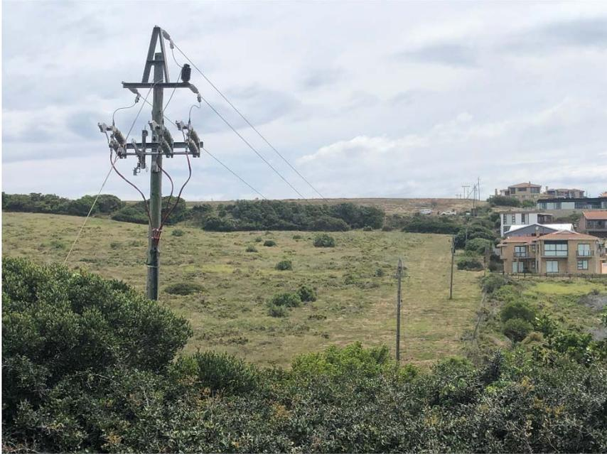
*Figure 1: Existing 11kV Overhead Line*
