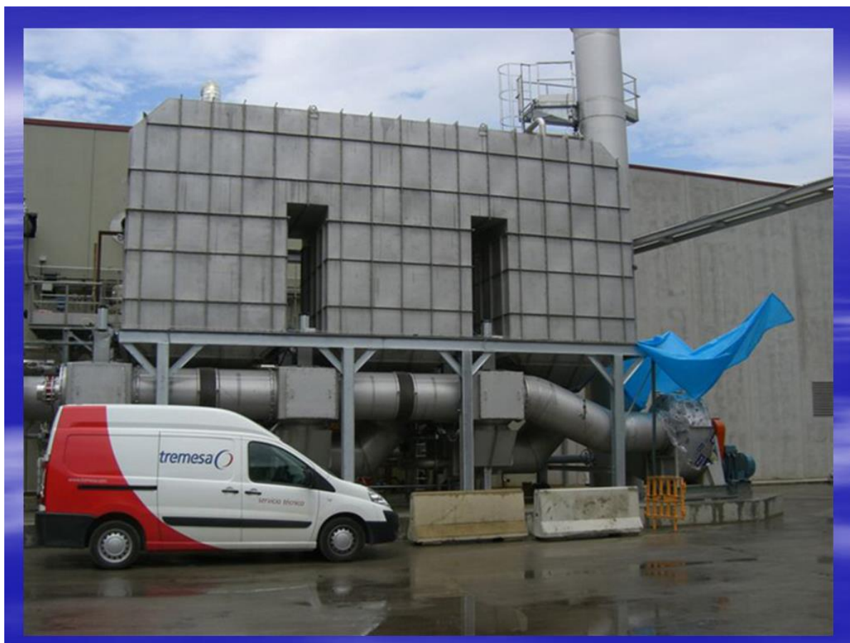
Figure 6: Regenerative Thermal Oxidiser (Tremesa, 2019)
