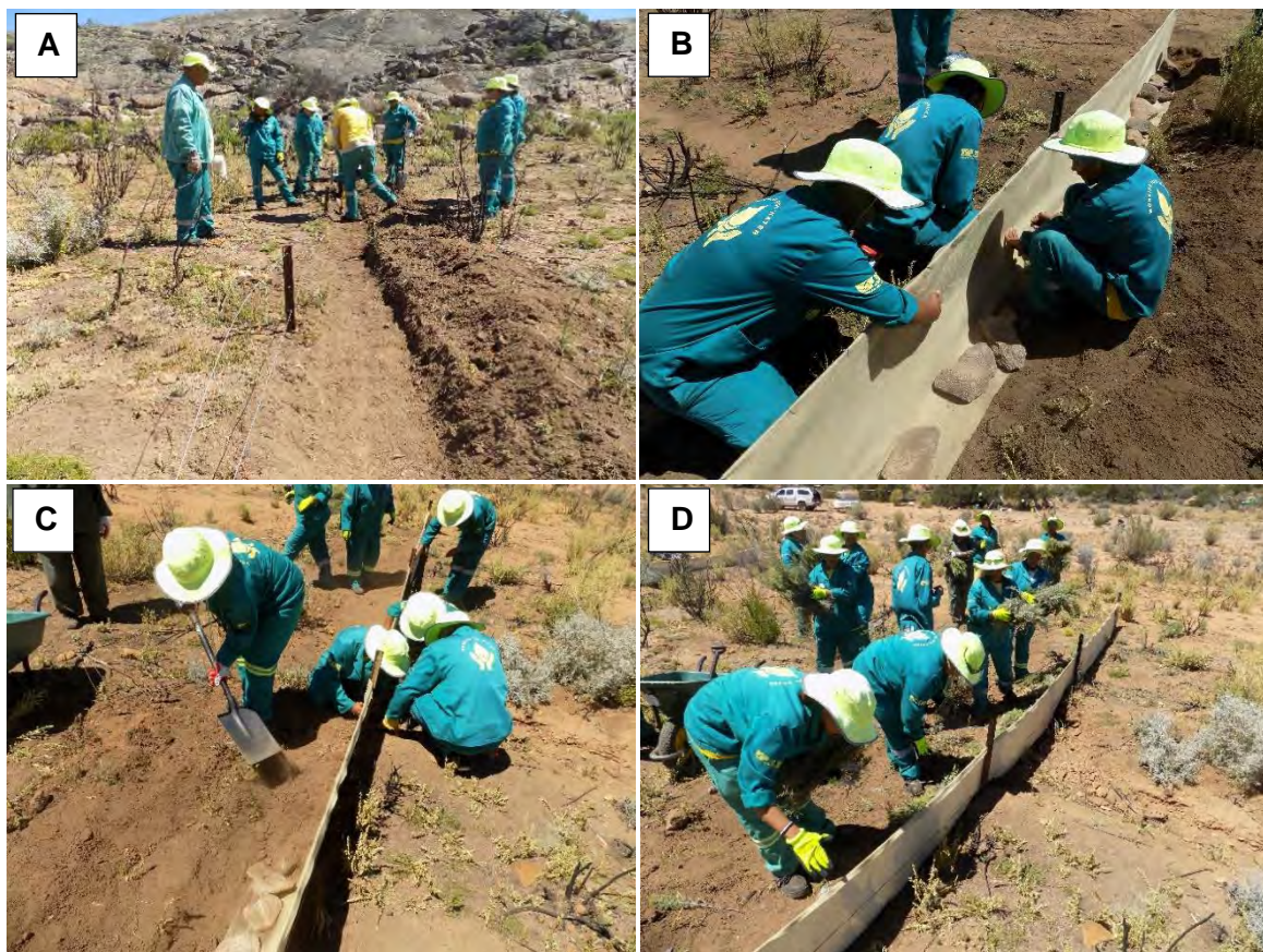
Figure 18. Installation of the soil erosion control fence. A: Installing the standards and wires and preparing the trench. B: Fitting the geotextile, tying it on with wire. C: Filling in the trench over the geotextile. D: Applying a mulch against the completed fence (Photos courtesy Ken Coetzee).
