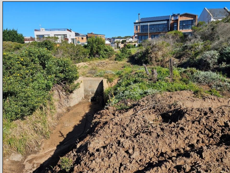
Figure 11: Existing Municipal stormwater outlet with headwall at the position where the entrance is proposed on property.
