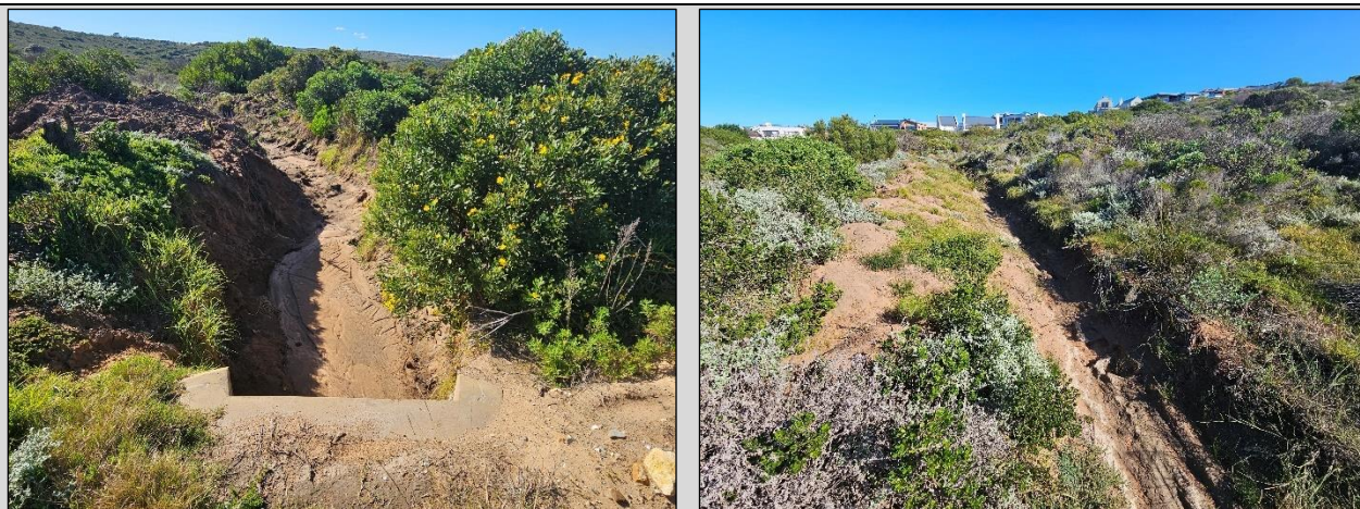
Figure 12: Existing stormwater headwall outlet & earth channel maintained traversing the property, maintained by the Municipality.
