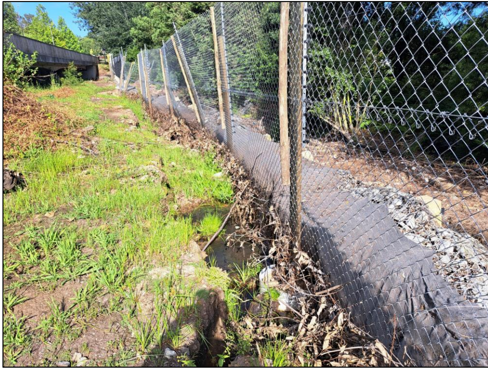
Figure 7: Channelled flow between the partially displaced gabion wall and the elevated riverbed along the western alignment of the fence
