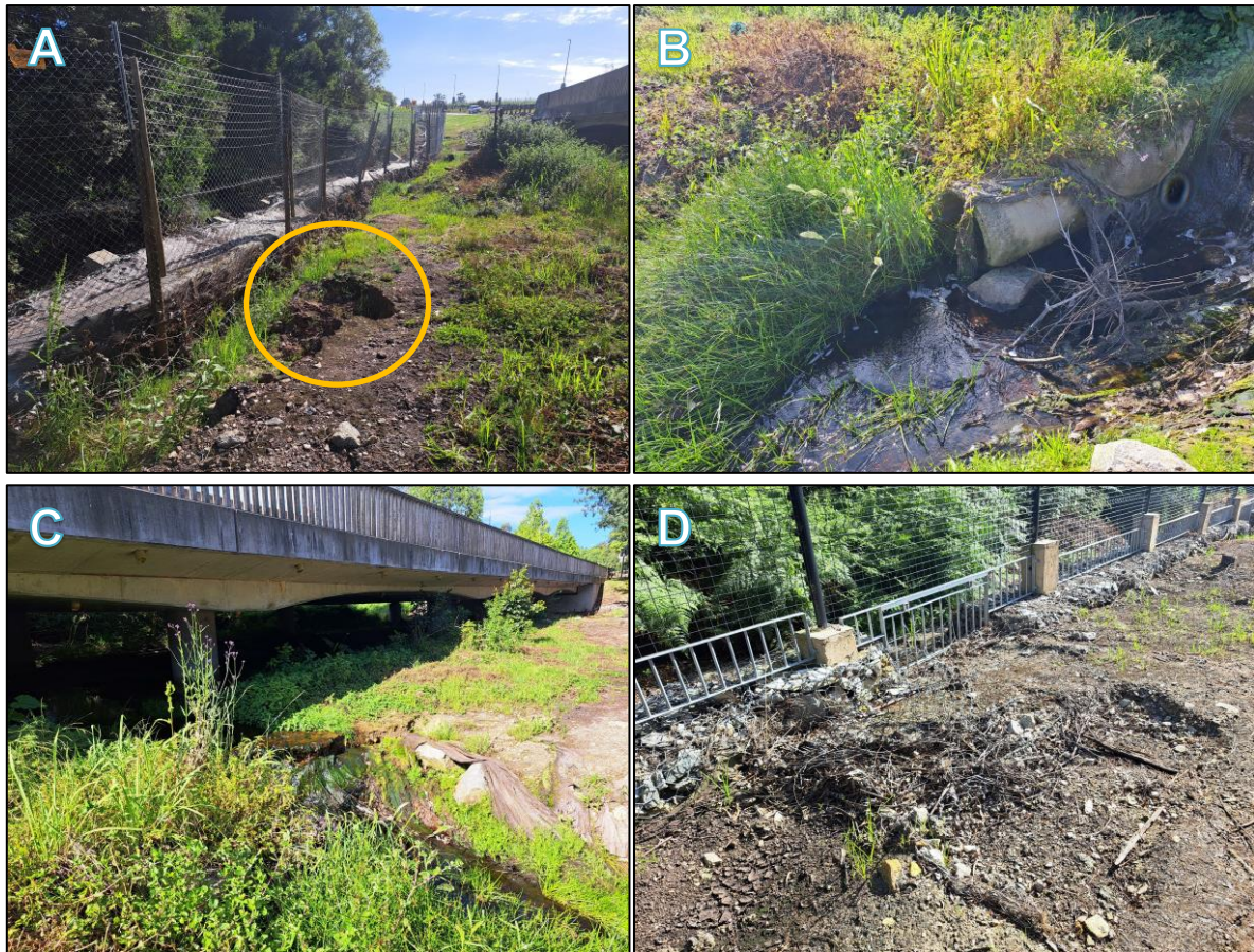
Figure 9: Photographs showing signs of erosion upstream of the fence (A); erosion around a culvert beneath the bridge, most likely caused by more channelised flow through gaps in the gabion wall (B); partial undermining of the concrete slab beneath the bridge (C); and intact gabions along the eastern alignment of the fence – slightly elevated above the level of the riverbed (D).
