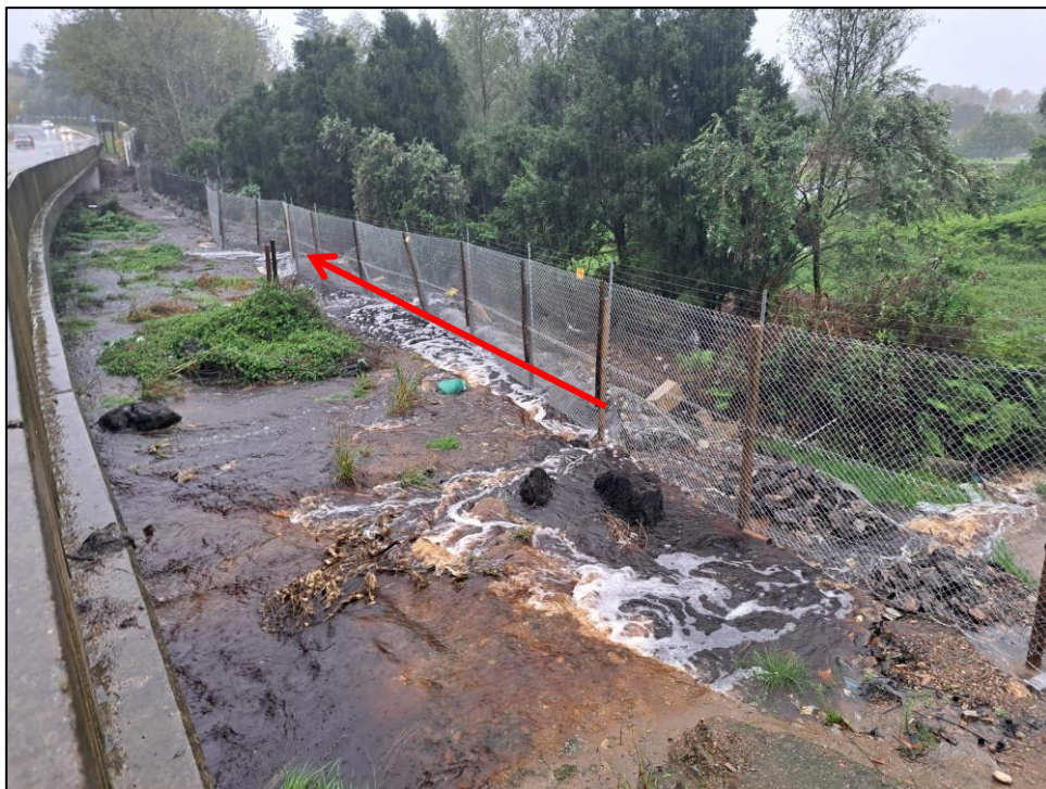
Figure 8: Photograph taken during a heavy rainfall event (4 June 2024) which shows the displaced gabion along the western alignment and channelled flow in between the gabion wall and the elevated riverbed (red arrow) toward a gap in the gabion wall.
