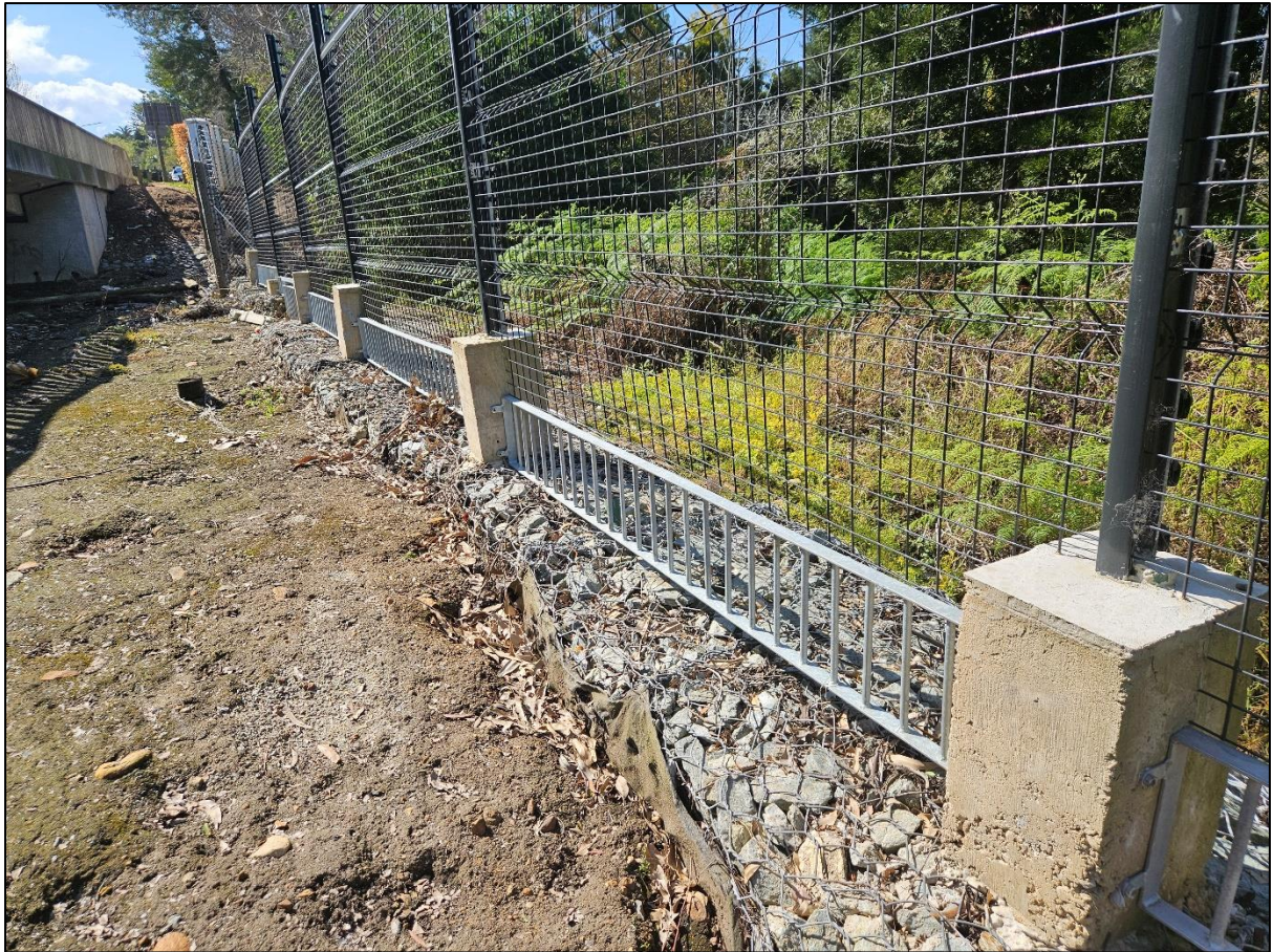
Figure 5: Exposed Gabions/Reno Mattresses and foundation of existing fence to be removed and replaced according to engineering design.
