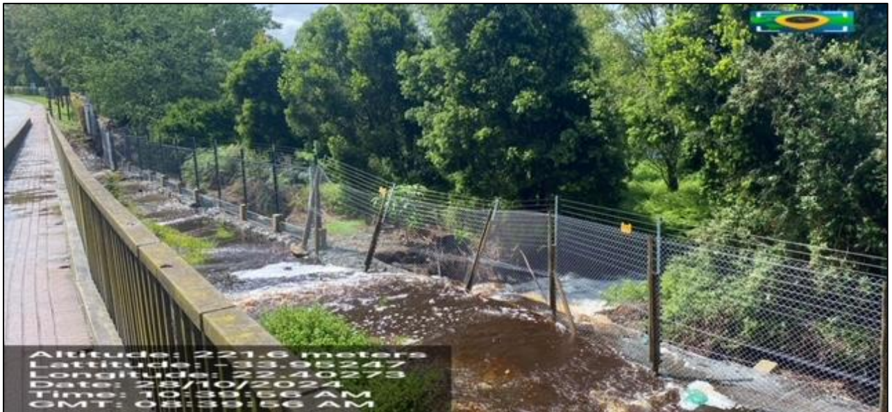
Figure 3: Portion of the failing fence damaged by waterflow (existing gabions/reno mattresses below water level during high flow).
