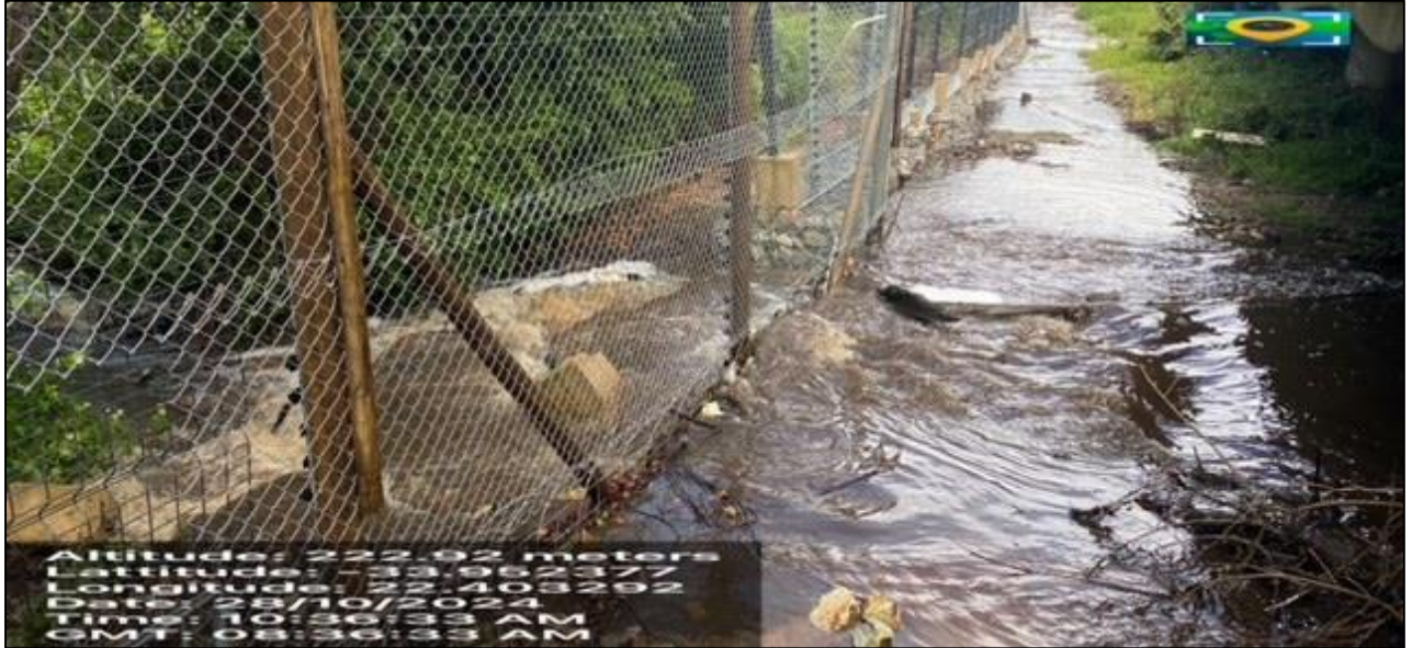
Figure 1: Portion of the fence erected on existing gabions/reno mattresses.
