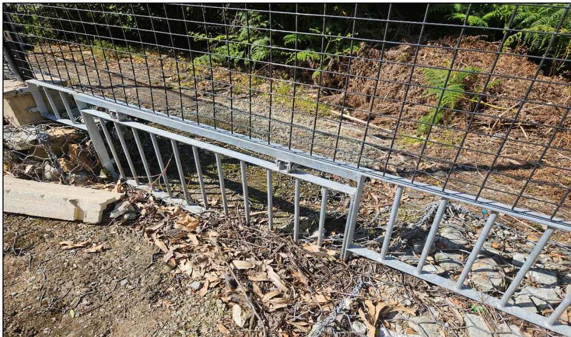
Figure 4: Existing Fence with unsustainable movable bottom section that is too narrow.
