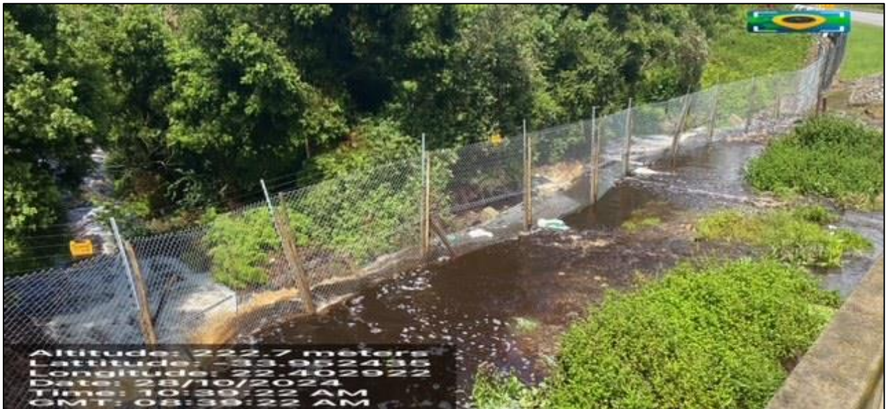
Figure 2: Portion of the fence where existing footings are covered during flow (view taken from bridge).
