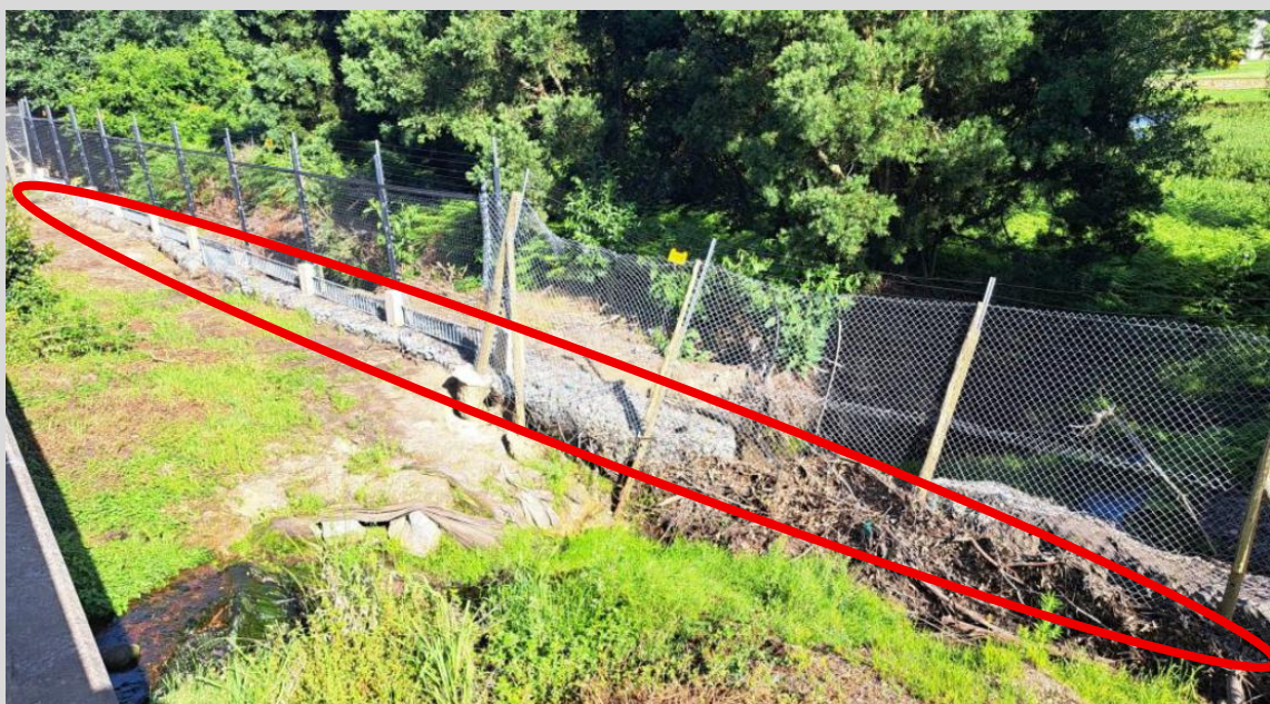
Figure 4: Indication of stabilising materials to be removed and lowered to create a more natural watercourse bed.
