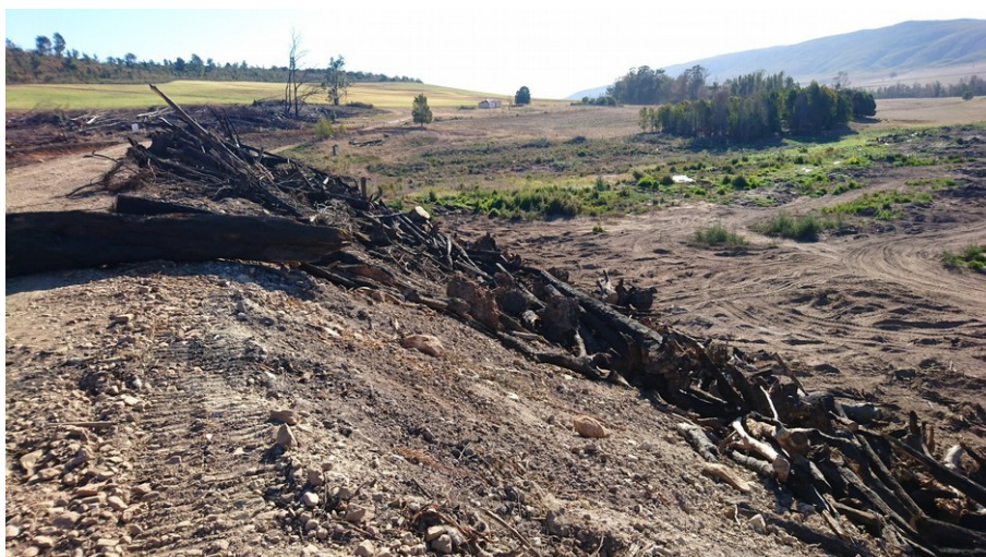
Figure 3: Downstream slope with tree stumps
