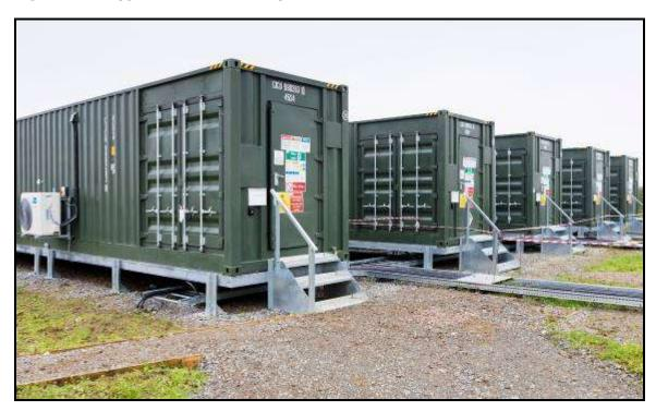
Figure 1.3: Example of BESS located in storage containers
