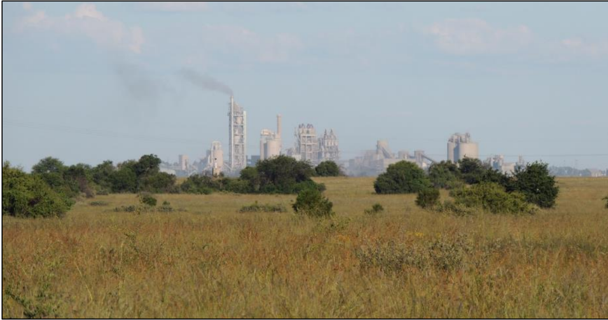
Figure 7. Zoomed photograph of the Lichtenburg LaFarge Cement Factory that forms a background view to the development areas.
