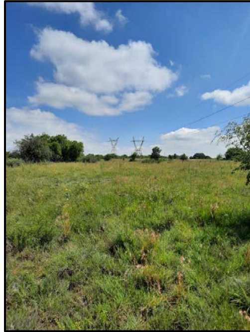
Figure 7.2. Powerline in the study area.
