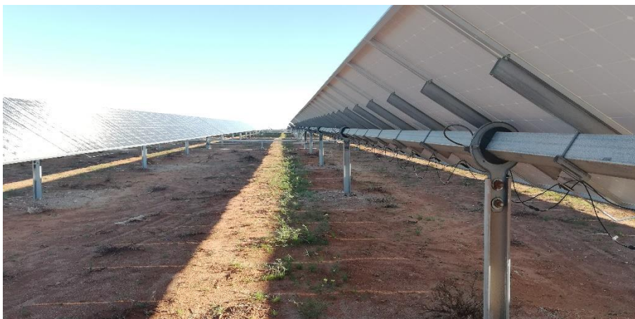
Figure 8: Showing vegetation re-establishing along the driplines of the arrays within weeks after installation.
