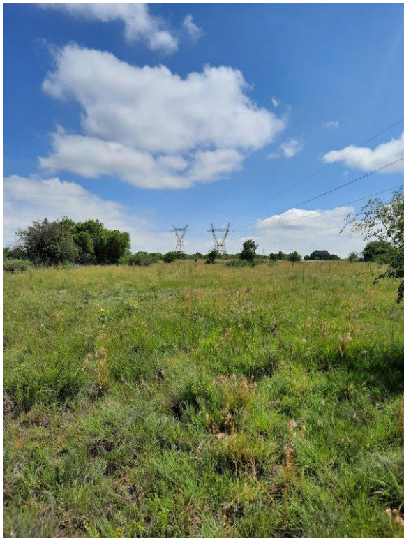
Figure 33: Existing powerlines traversing the Aristida PV site.(van der Walt, 2022).
