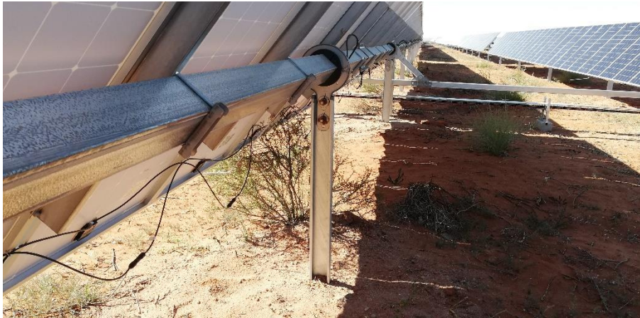
Figure 7: Completed racking and assembly showing vegetation remaining intact beneath the modules.
