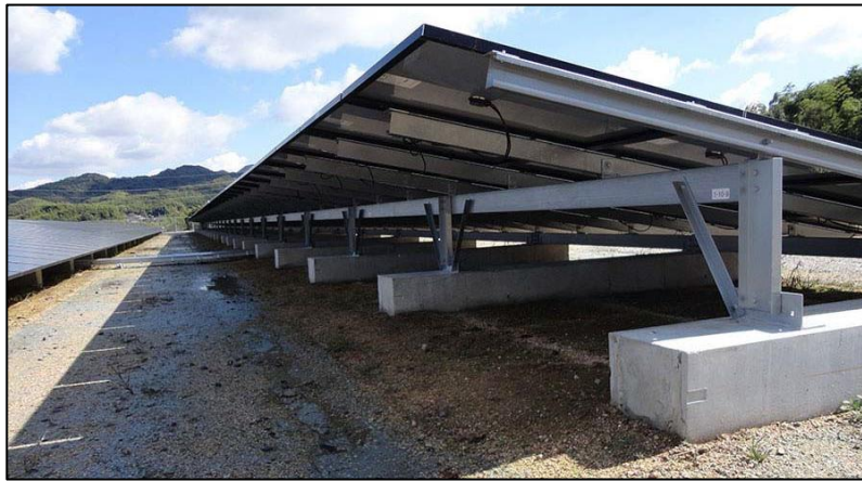
Figure 4: Cast Concrete Foundation
