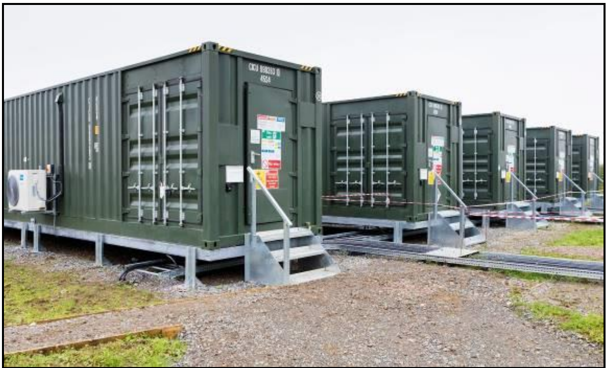
Figure 1.3: Example of BESS located in storage containers
