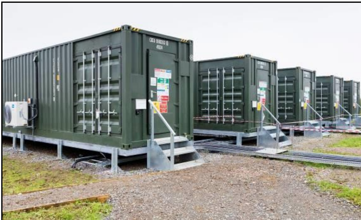
Figure 1.3: Example of BESS located in storage containers
