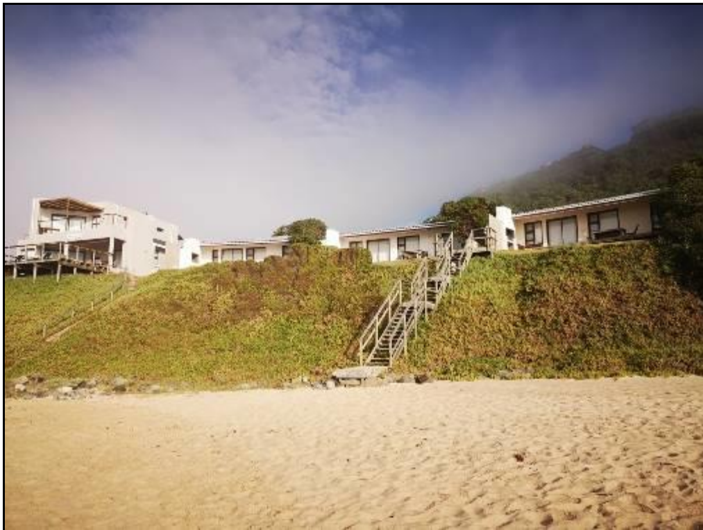
Photograph 1.9: Three units overlooking the beach that will be redeveloped
