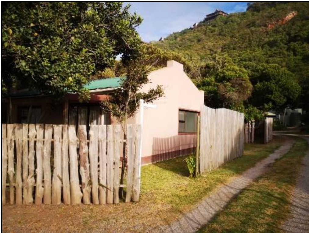
Photograph 1.11: brick and mortar unit
