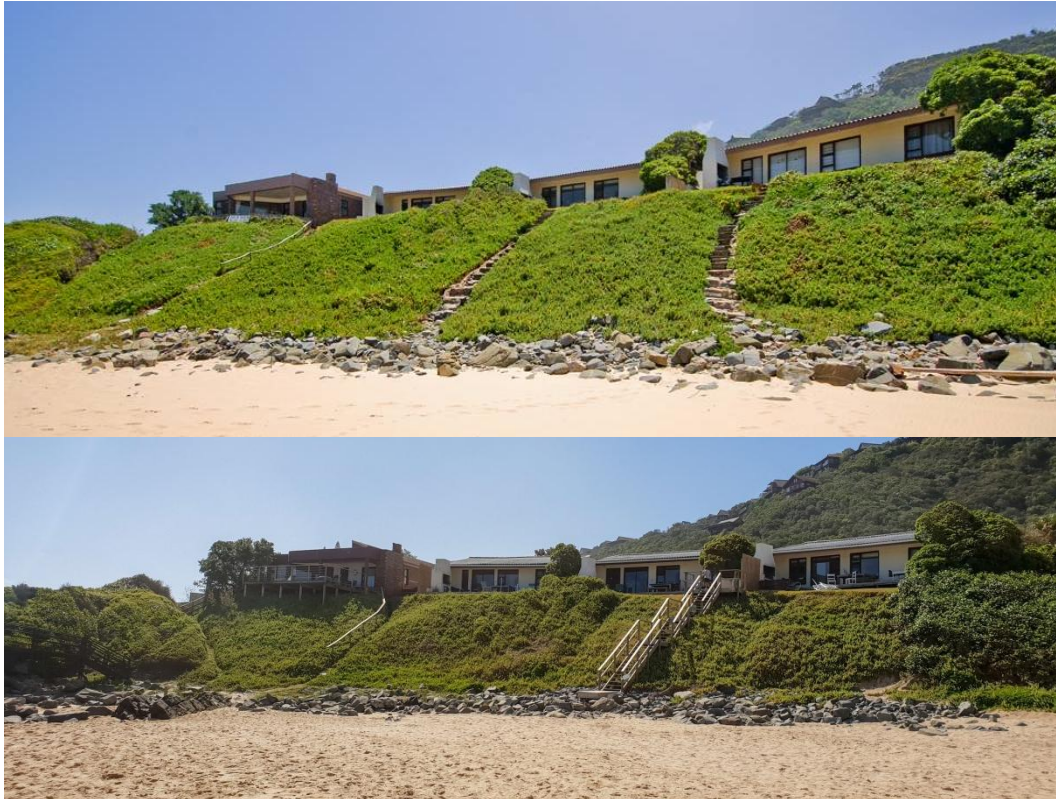
Figure 9: The vegetation density on the seaward slope appears to have improved following replacement of the older beach access pathways (top, archrock.co.za) with an elevated wooden staircase (bottom, twitter.com @Arch_Resort)
