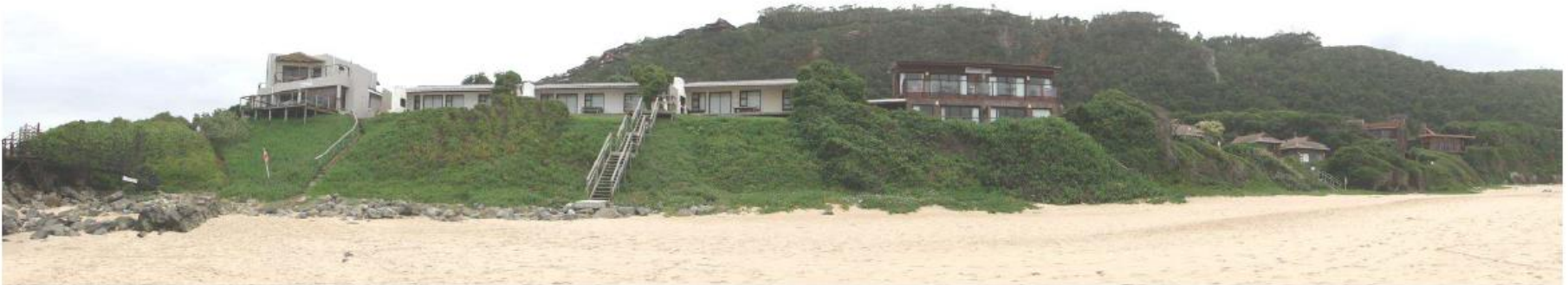
Photo 15: North-facing contextual view of the property from beach.
