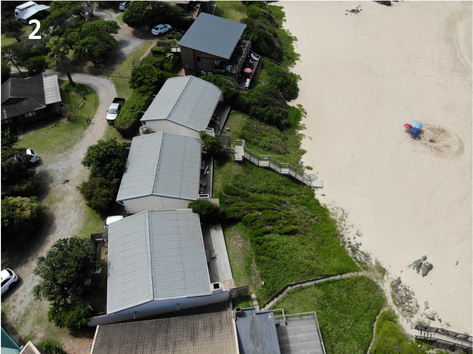
Photos 2: View from west to east of the three sea facing units.
