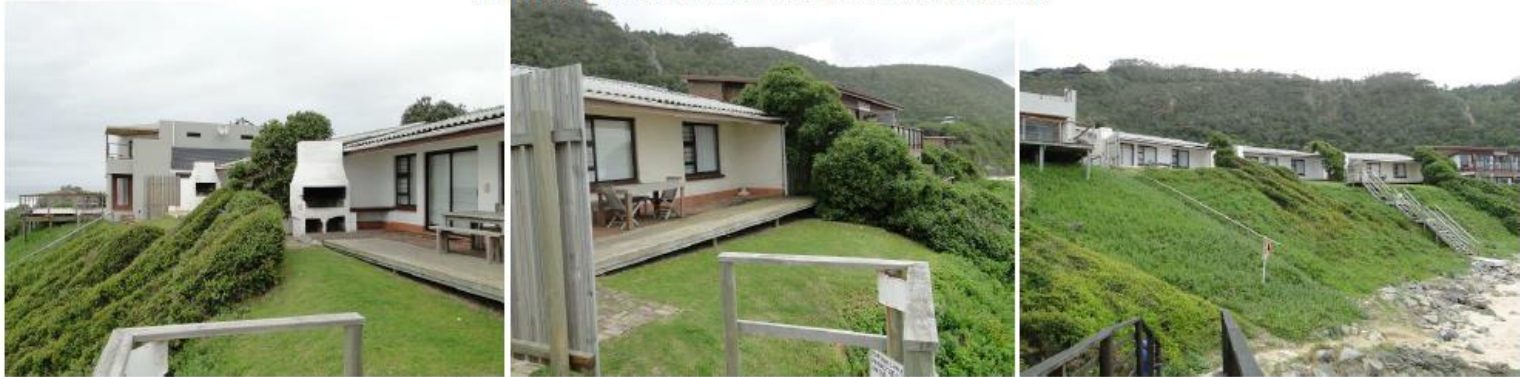
Photos 12,13,14: Three units and timber decking leading onto the beach.
