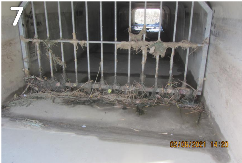
Photo 5 & 6: Completed access road over tidal channel. Photo 7: Culvert with access control, shows height of water moving through at high tide. Photo 8: Exposed mudflats of the tidal channel showing improved water quality and habitat.
