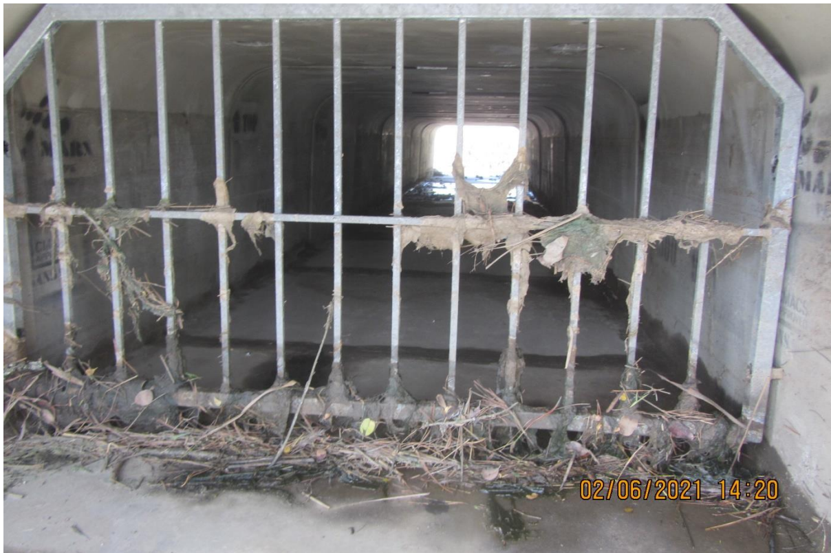
Photo 3: Evidence of improved tidal movement through the culvert
