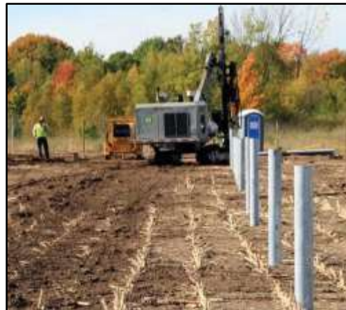
Figure 5: Driven/ Rammed Steel Pile
