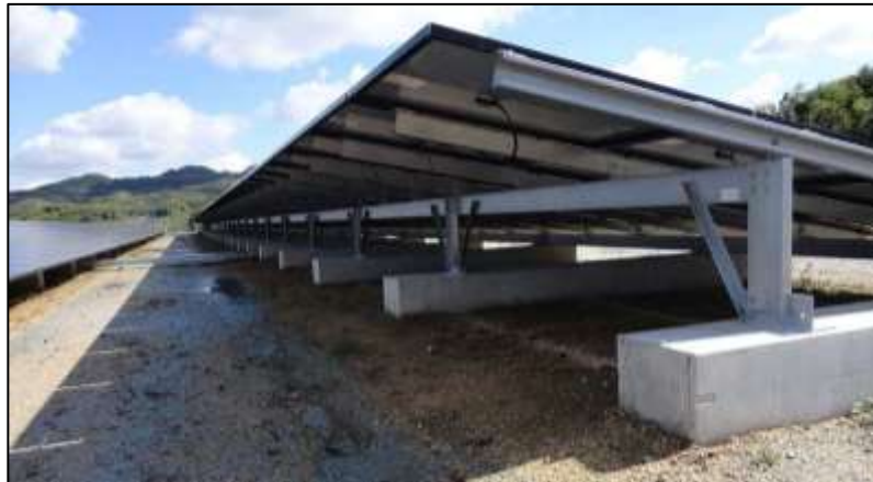
Figure 4: Cast Concrete Foundation
