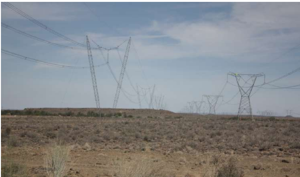
Figure 4. Views of the Eskom transmission lines traversing the site.
