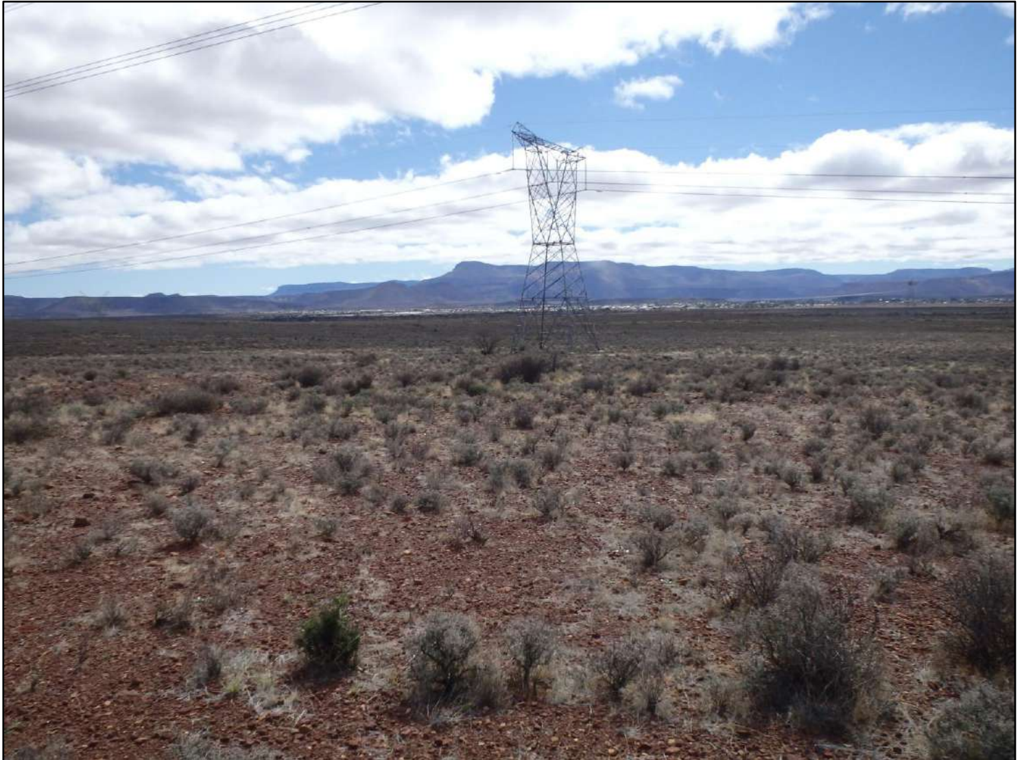
Figure 4.9: Contextual Images of grid connection corridor
