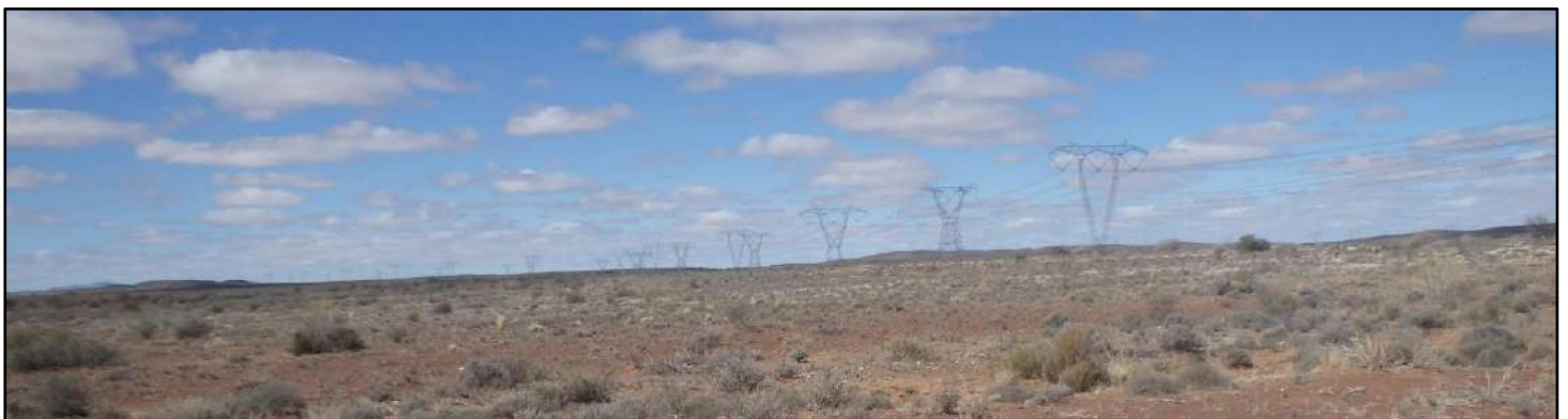
Figure 4.5: Contextual Images - Existing grid connection along proposed grid alignment
