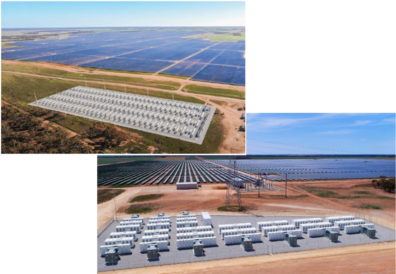
FIGURE 2.3.1.1 – Images of Typical BESS Systems Servicing Renewable Power Farms
