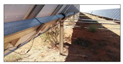
Figure 9: Completed ramming and assembly showing vegetation remaining intact beneath the modules.
