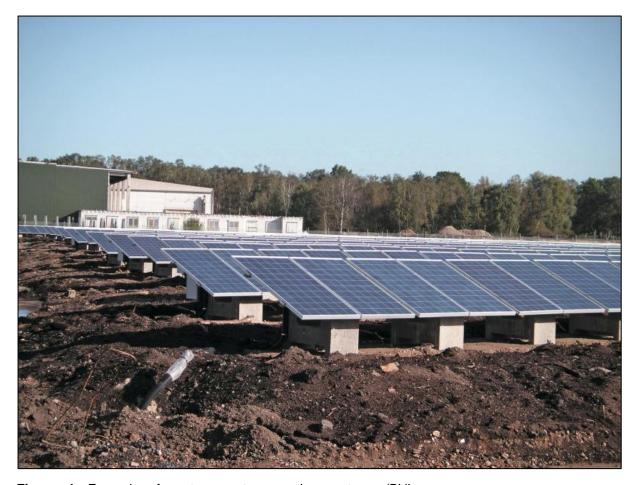
**Figure 4:** Example of cast concrete mounting systems (BVI International 2023)
