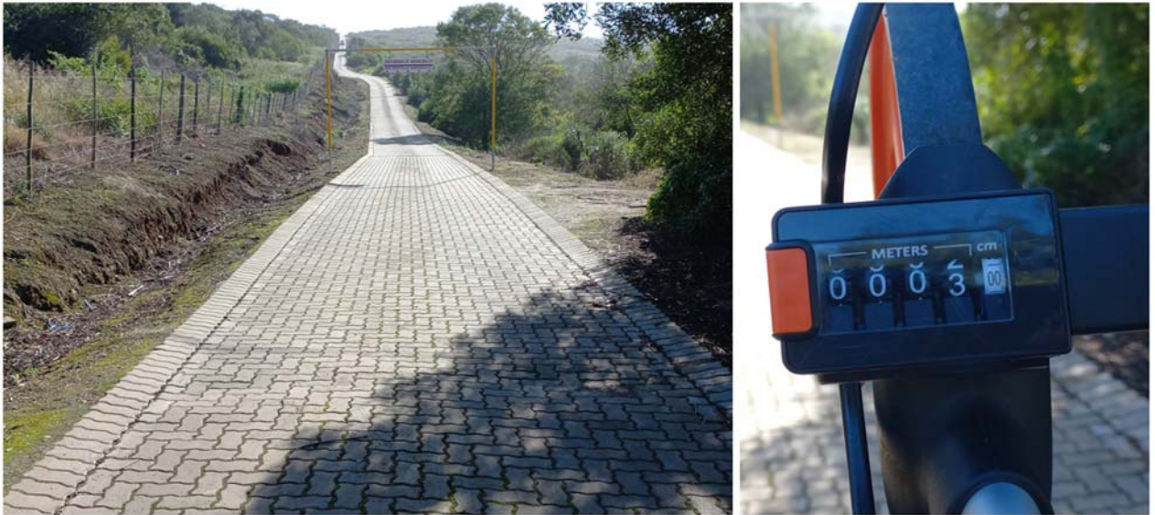
Figure 8-5 - Existing Servitude Road
