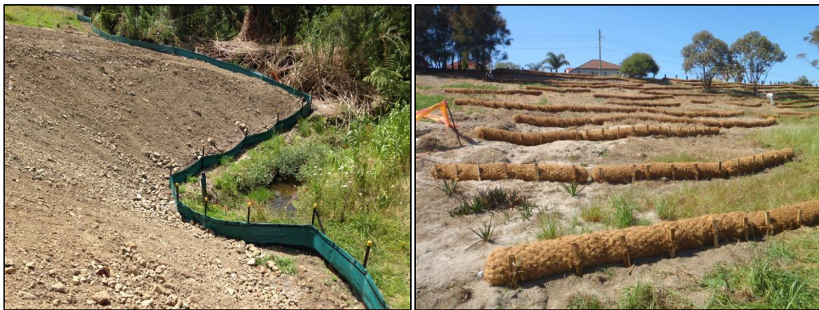
Figure 6: Examples of silt fences (left) and coir logs (right) used to trap sediment mobilised from steep slopes.
