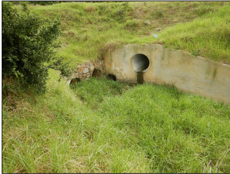
Figure 5: Stormwater inlet into the watercourse.
