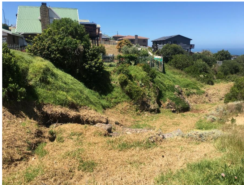
Figure 5: Slope erosion presents a threat to property adjacent to watercourse.
