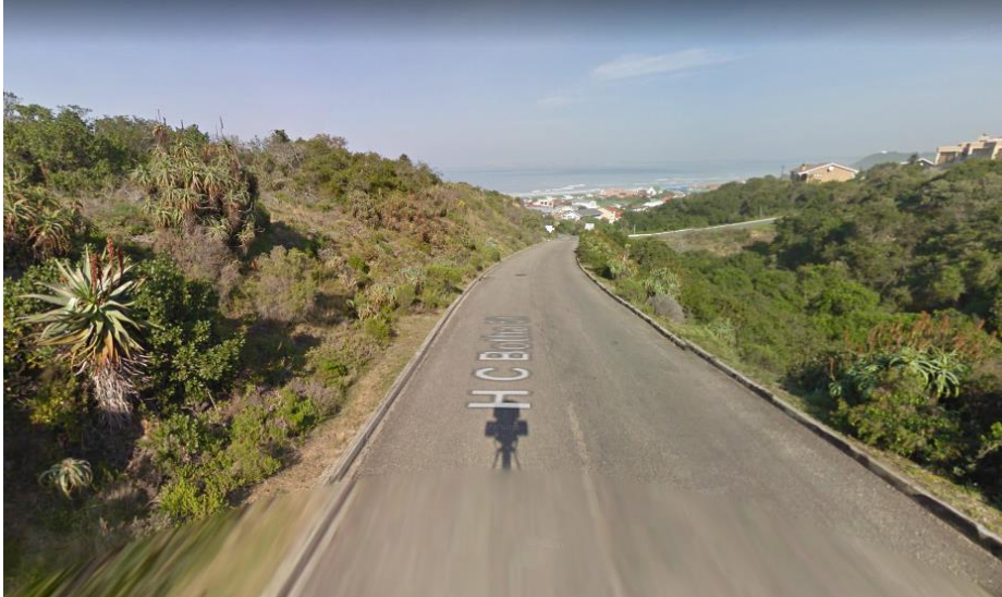
Figure 16: South-western view along HC Botha street at proposed access point indicating very good sight distance in the vertical and horizontal alignments.
