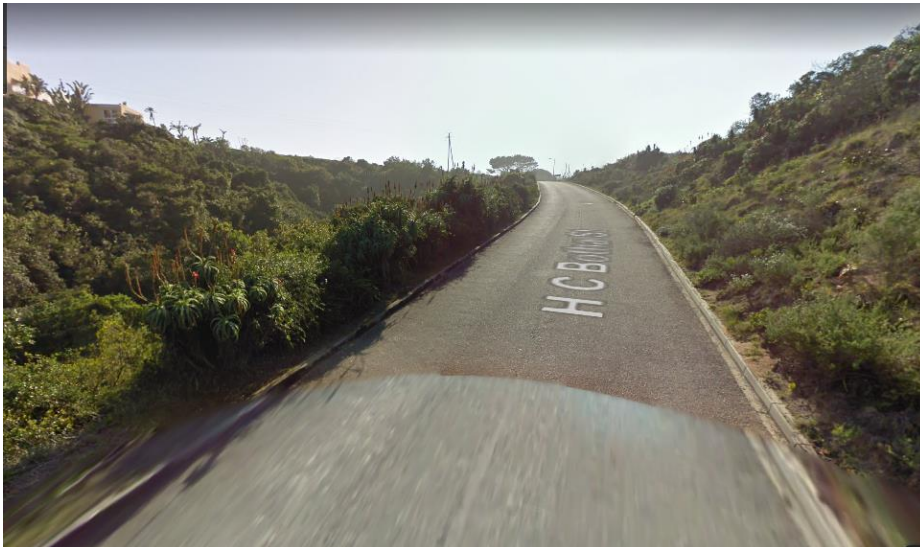
Figure 15: North-eastern view along HC Botha street at proposed access point indicating very good sight distance in the vertical and horizontal alignments.
