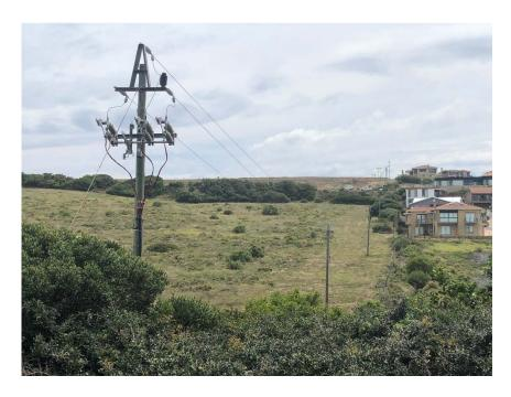
Figure 1: Exiting 11kV Overhead Line
