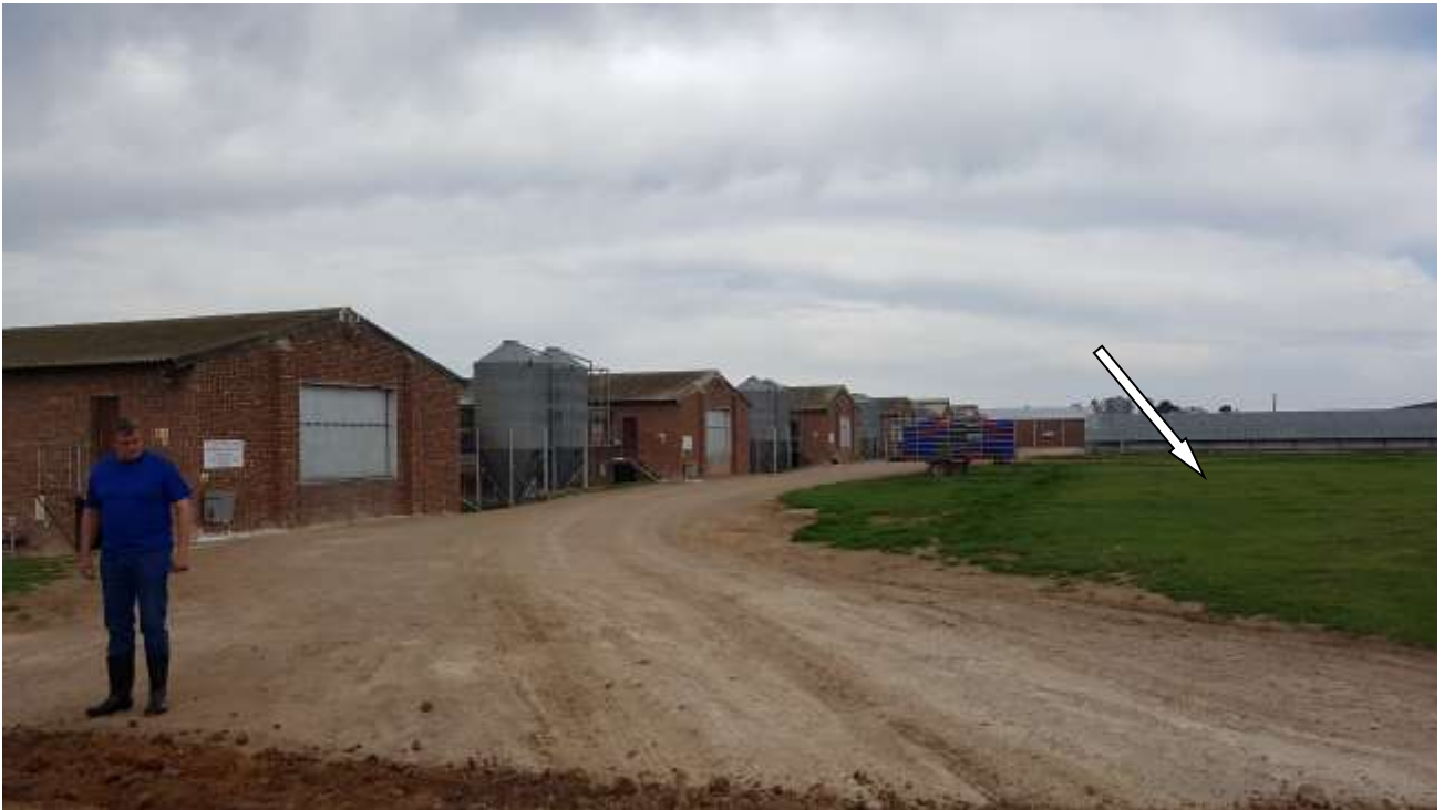
Figure 5: Existing lay houses on the left of image (6) and two (2) lay houses constructed without prior EA on the right side on the kikuyu lawn. Arrow points to the location of the proposed two (2) new lay houses and evaporation pond.
