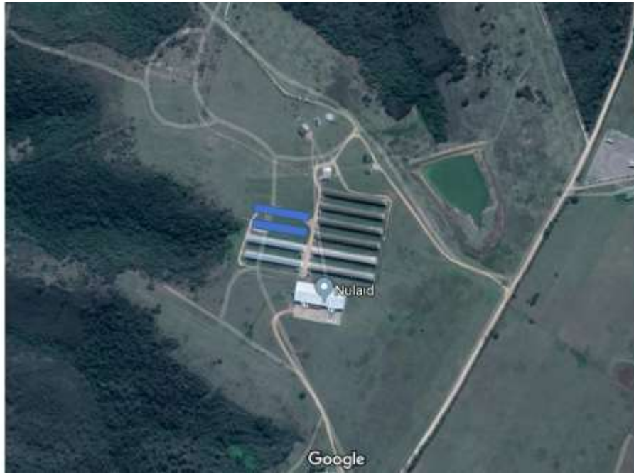
Figure 1: An aerial view of the current facilities associated with Thornhill Egglund and the two proposed houses (blue rectangles)
