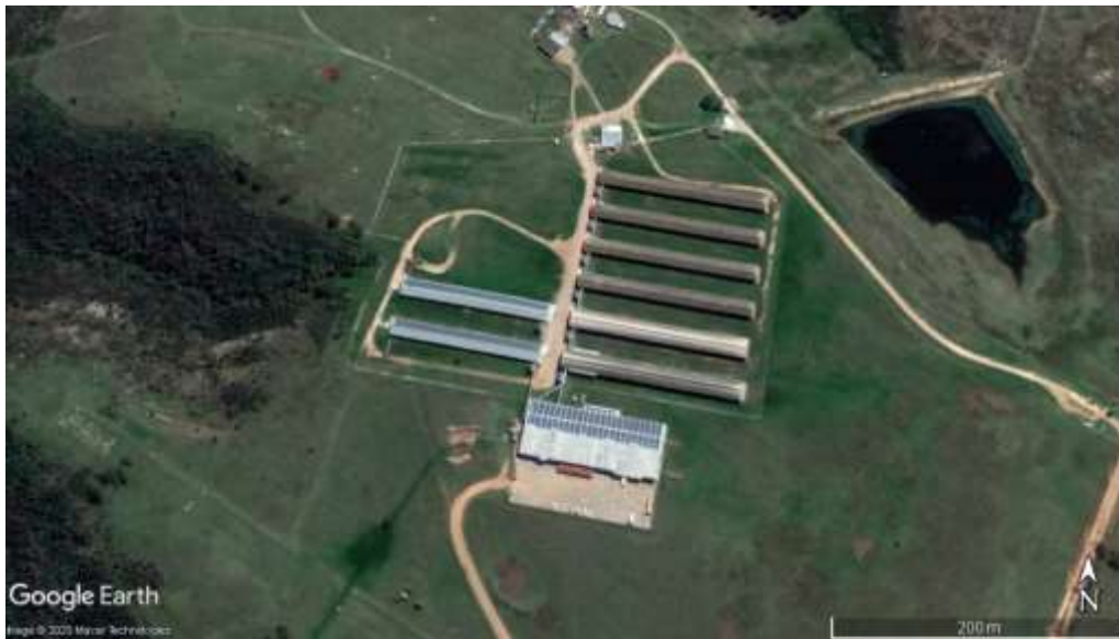
Figure 1: An aerial view of the facilities associated with Thornhill Eggland
