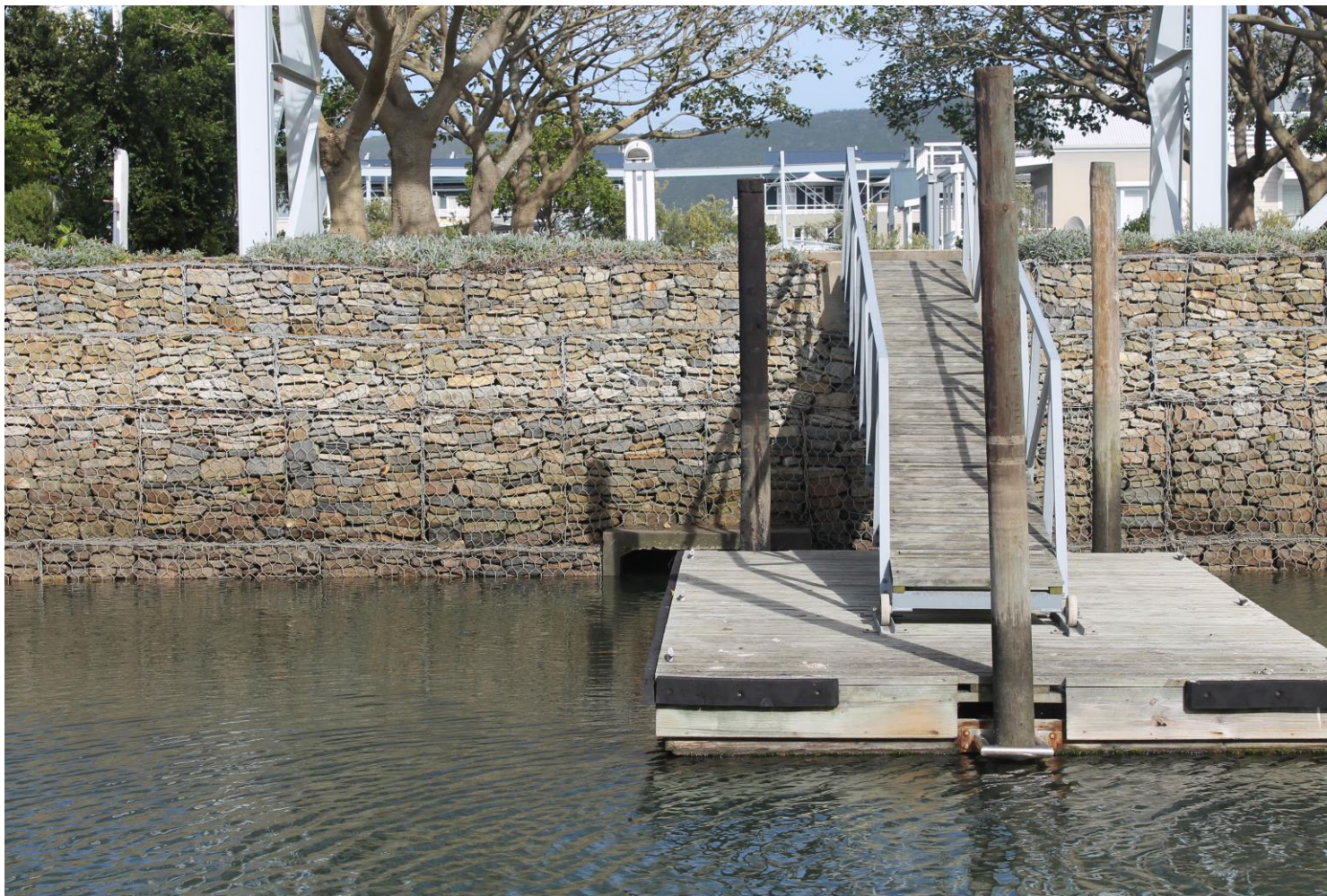
Figure 15: Floating jetty with movable ramp accommodating tidal fluctuations (fixed with poles that are inserted into the substrate).
