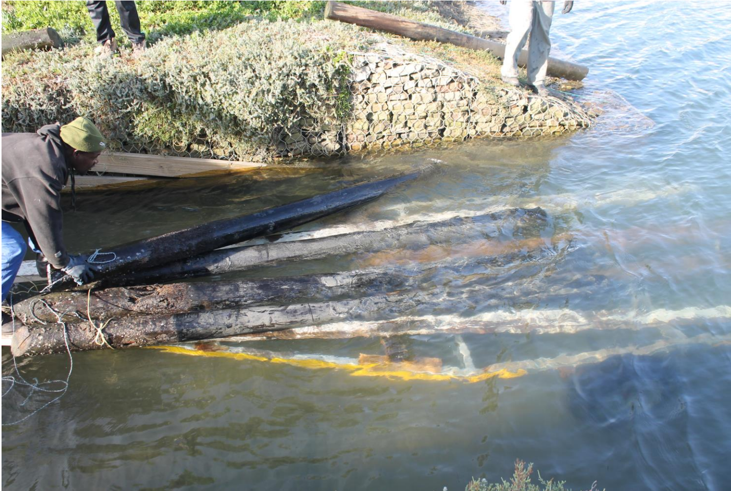
Figure 16: Example of how jetty poles are recovered from the water after being removed from the substrate.
