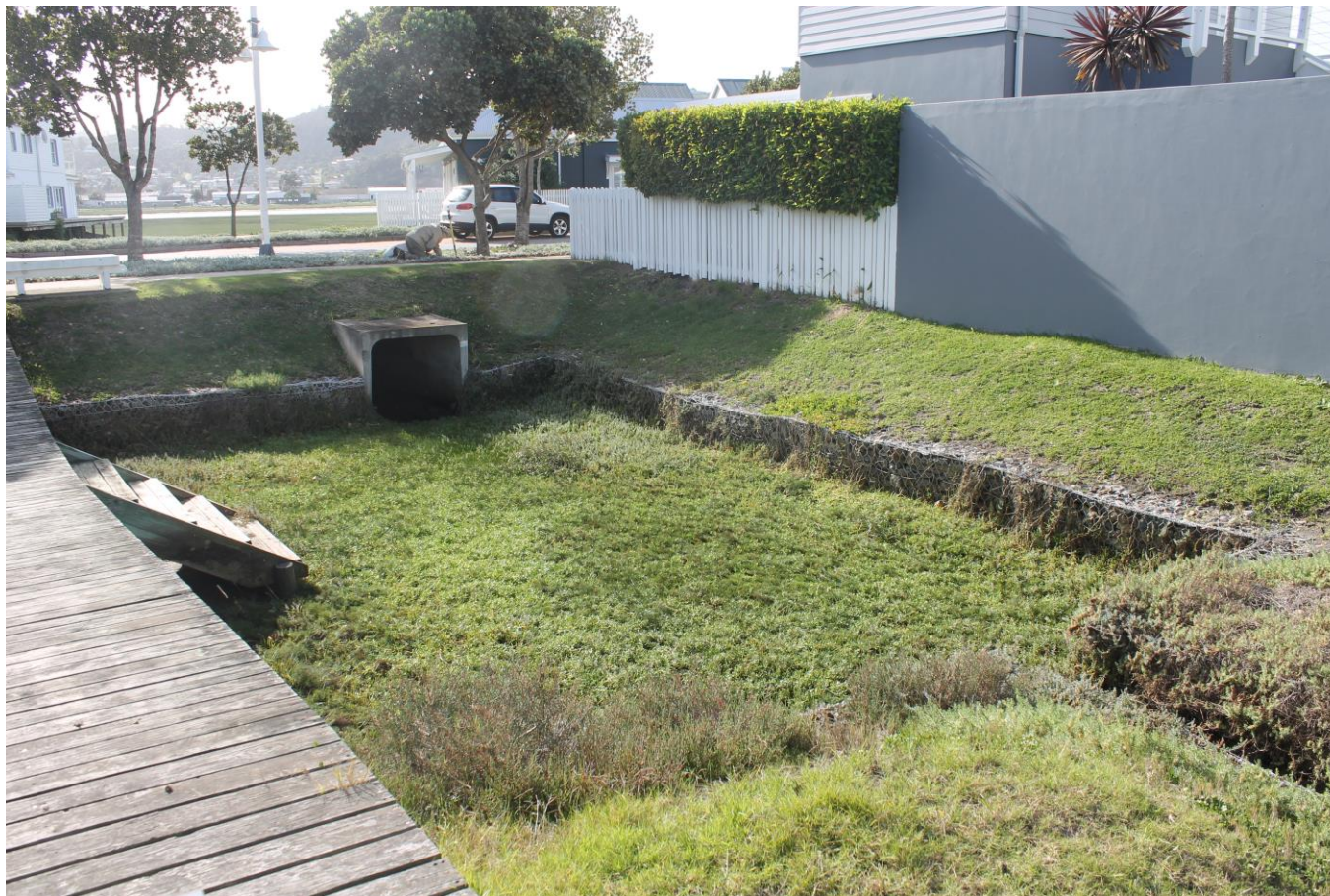
Figure 9: Example of stormwater stilling basins found within the open space (eco-belt) with existing gabions extending into the soil, covered by vegetation (that must be removed and excavated for maintenance purposes when it is required).
