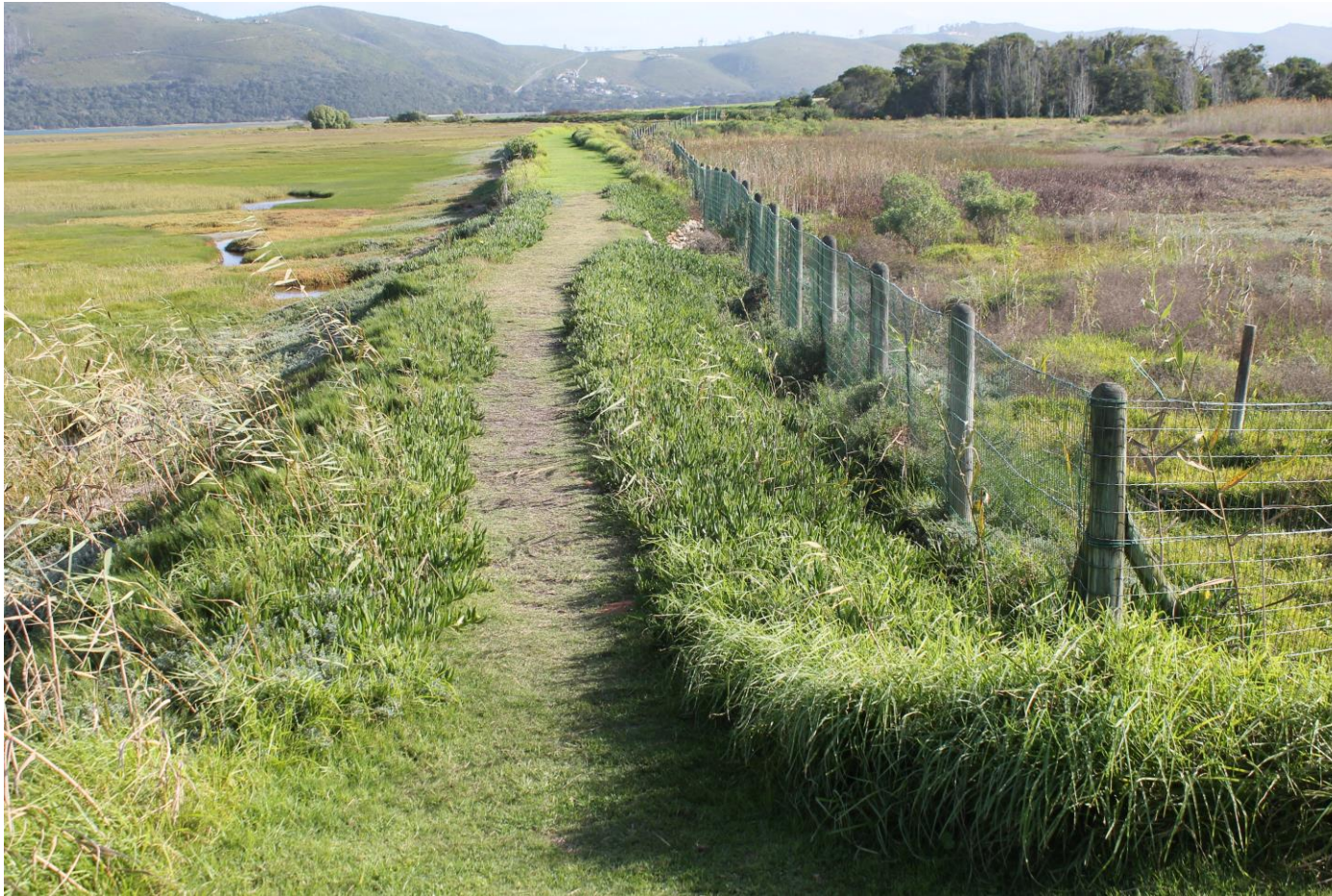
Figure 13: The artificial seawall is visible as a berm used for hiking/cycling separating the reed bed (right-side of the image) from the estuary (left side of the image).
