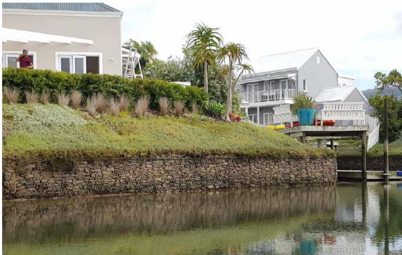
Figure 7: Example of existing gabions forming the stabilising edges of existing artificial channels (Nieuwoudth & Kie, 2018).
