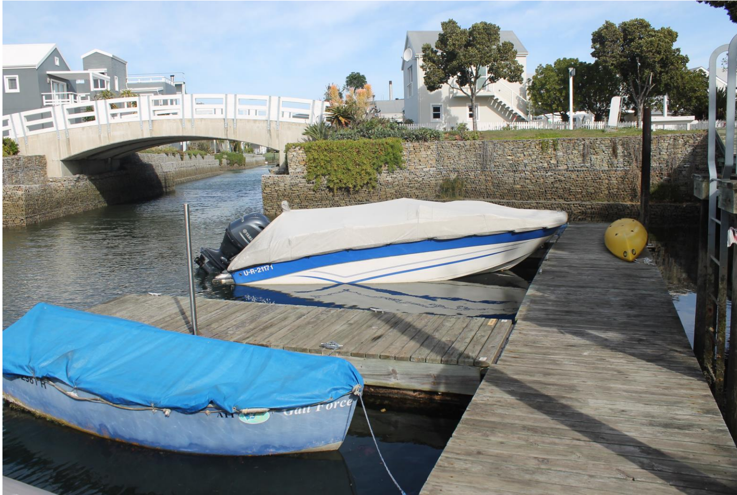
Figure 14: Floating jetties located within a designated mooring space (fixed with poles jettied into the substrate).
