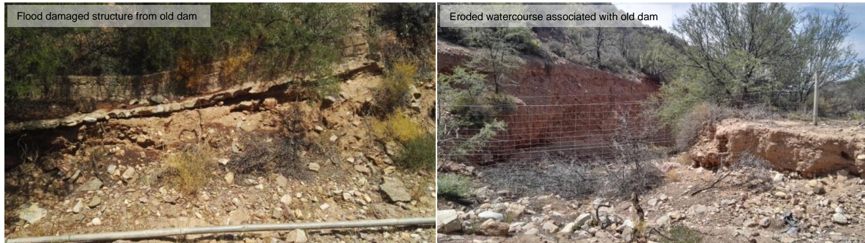
Figure 1. Photos showing construction of the new dam in progress and the finished dam as well as the spillway and channel constructed from the dam wall to orchards for irrigation. The old dam was washed away in floods with associated debris and erosion damage still visible in the basin downstream of the new dam.
