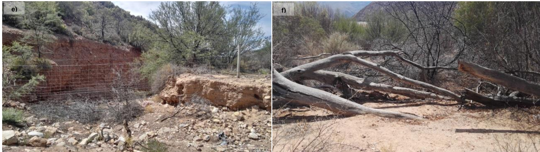
Figure 8. Photos from various points assessed along the watercourse including the area upstream of the dam with erosion of the banks and channel (a and b) and accumulated sediment in the river bed (c), part of the watercourse in relatively good condition that lies within the full supply level of the dam but hasn't been cleared yet (d); and, flood damage and erosion of the watercourse (e), along with sedimentation in areas (f) downstream of the dam wall.
