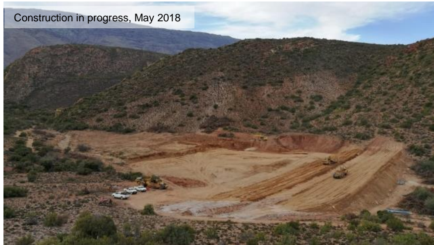
Spillway on west side of dam wall
