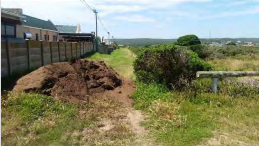
Figure 27: Berm created along Erf 2594 bordering Palinggat Resort to prevent vehicular access along the servitude.
