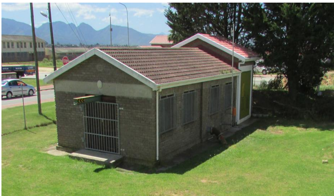
Figure 7: Existing pumpstation PWT-PS-01
