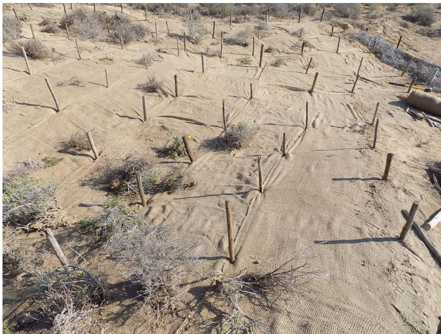
Figure 20. Example of how Soilsaver is fitted to the soil surface (Photo courtesy Ken Coetzee). Note holes to accommodate indigenous vegetation.
