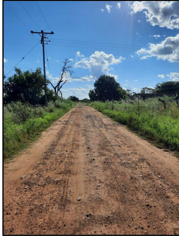
Figure 7.2. General site conditions in the study area showing existing infrastructure.
