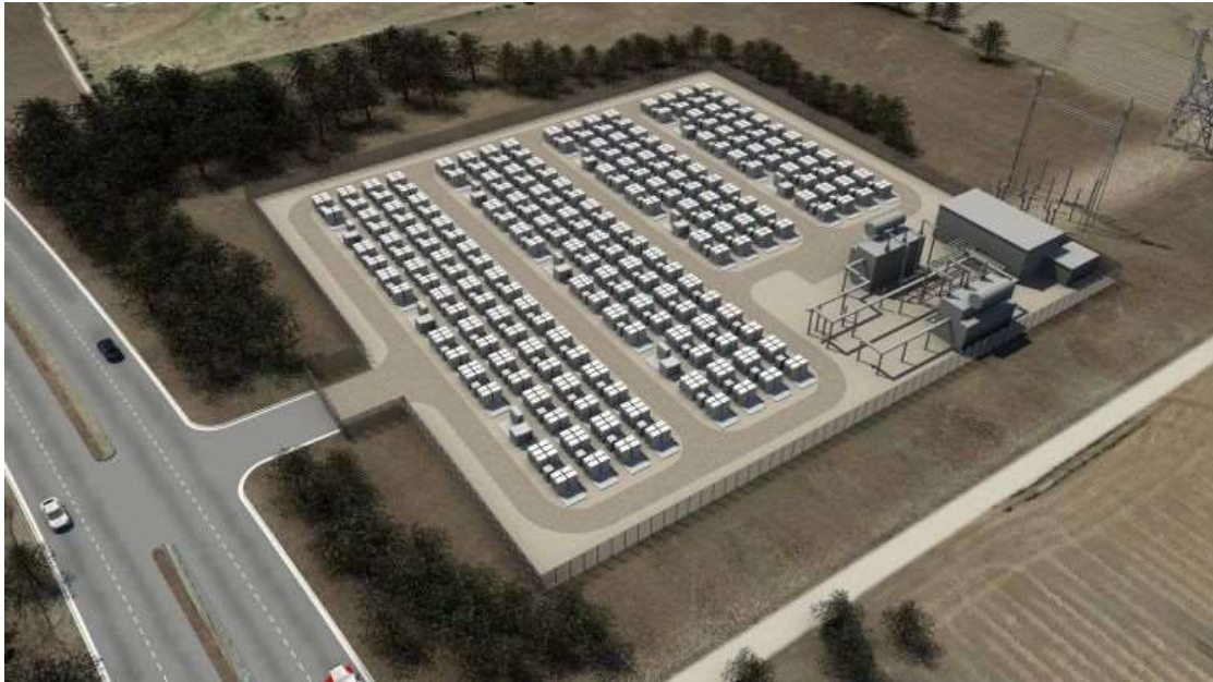
Plate 2.1: SolarCity's Tesla Battery Storage Facility, Hawaii. [Source: https://www.pv-tech.org/news/solarcity-picks-tesla-for-52mwh-of-dispatchable-solar-plus-storage-in-hawaii ]
