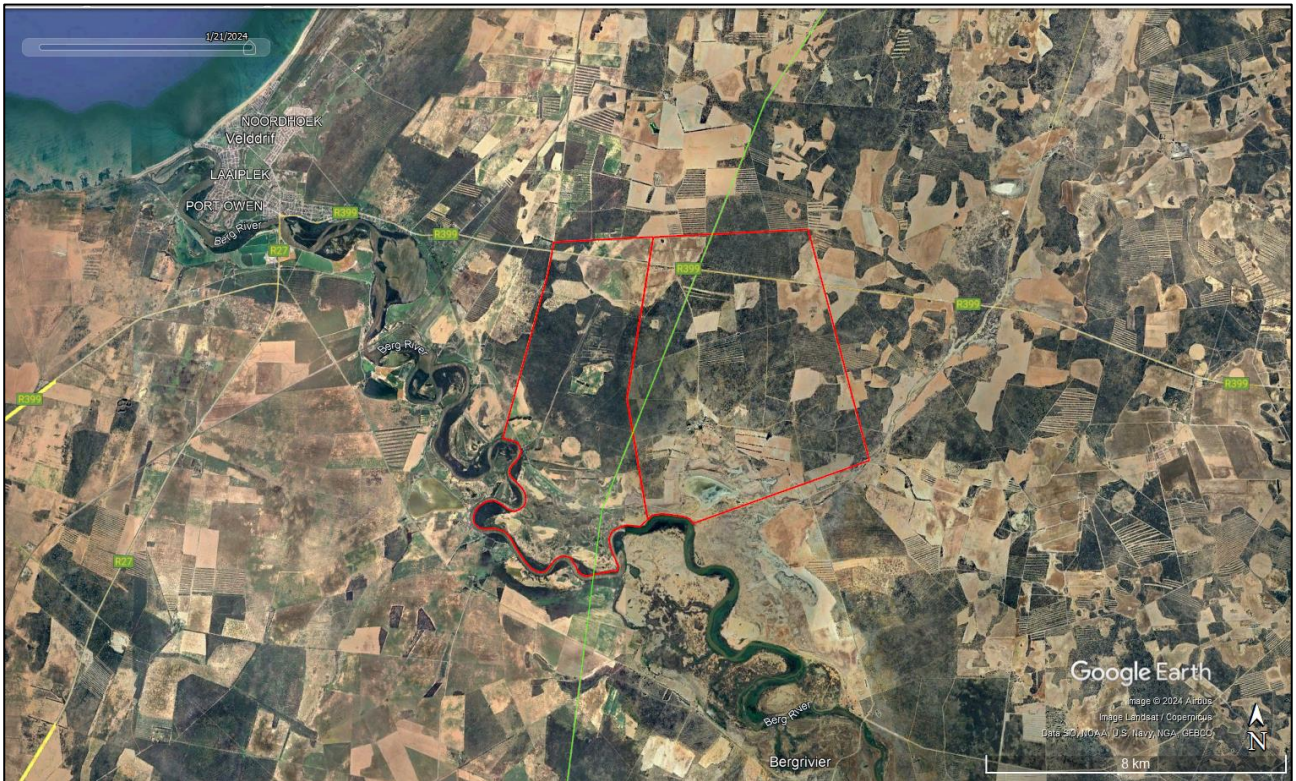
Figure 4: Aerial view of the study area (red polygons = affected farms) showing the landscape context and position of the existing Eskom HV powerline (green line).
